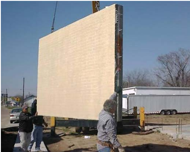
Figure 4. LGS system with a concrete in-fill being placed on site
