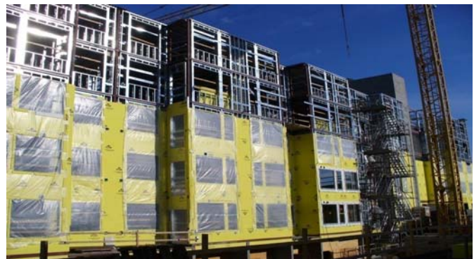
Figure 3. Assembling of LGS frames for high rise construction, West Town, 2007
