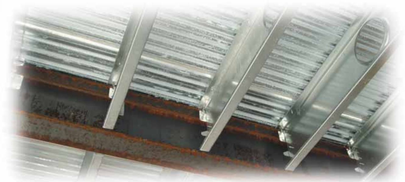
Photo illustrates SJCT Hanger. Bridle Hanger is an acceptable alternative.
